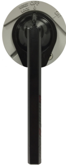
Figure 3: Main Disconnect Switch
